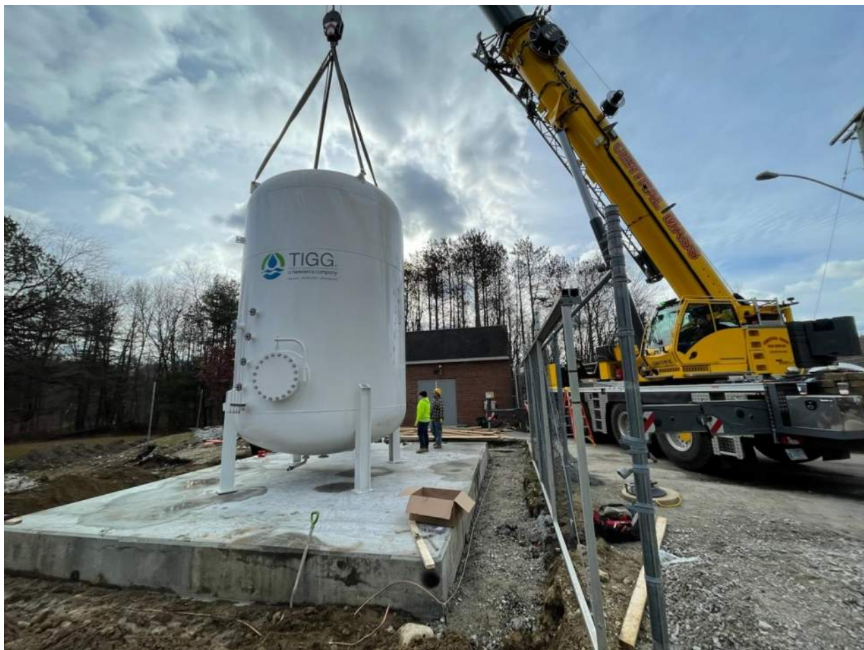
Photo 1: GAC filter vessels being installed in Dudley, MA. These filter vessels are 12-ft diameter and 24-ft tall for reference.
